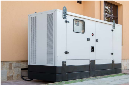
Engine / Generator starting
